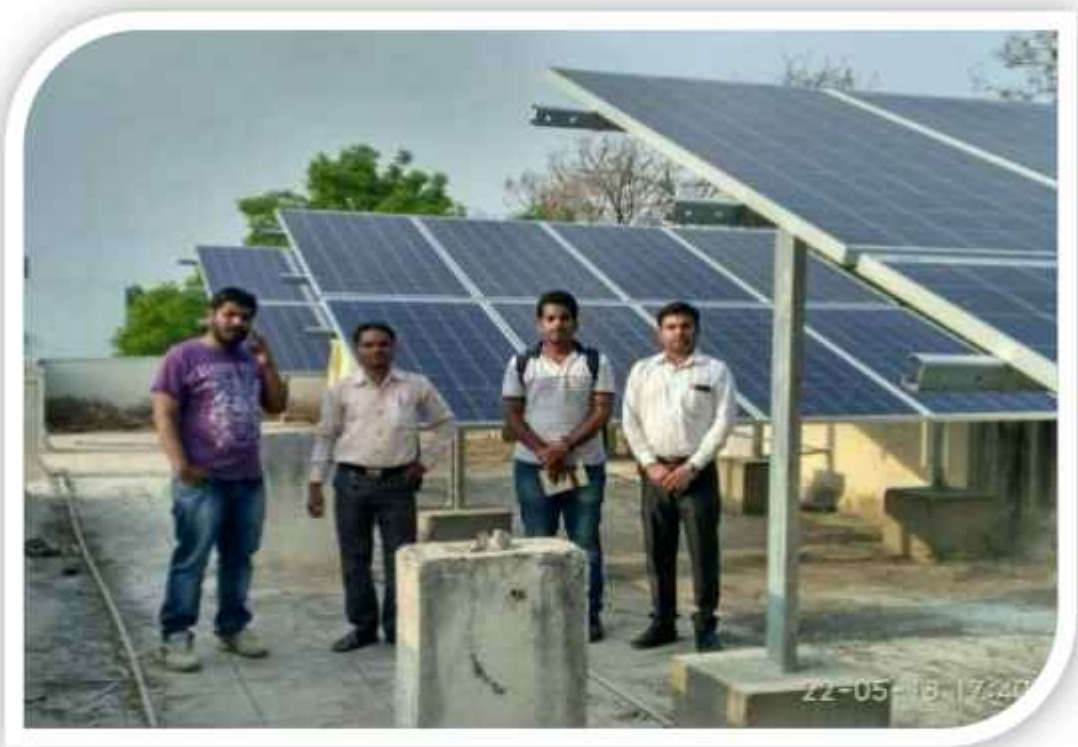
10 KW project Jain Solar at Girls Hostel
